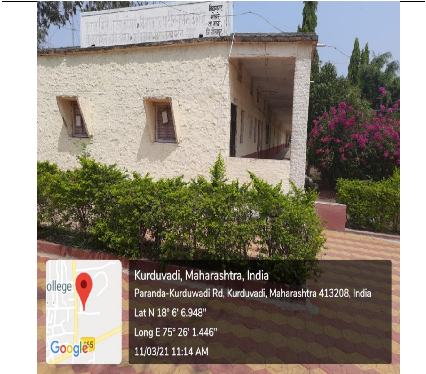
B. Building (Arts Commerce Building)
